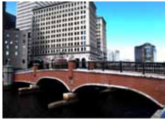
Weybosset Bridge today
